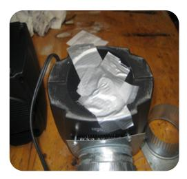
Heaters have a safety switch on bottom which has tape over. If tape comes loose the heater may turn off so make sure tape is secure.
