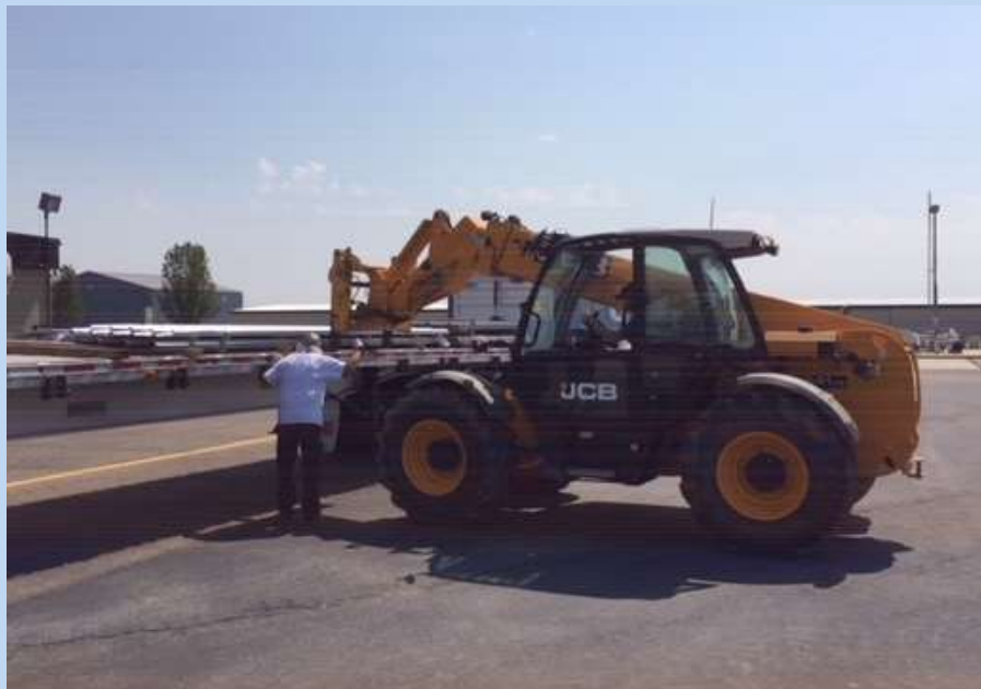
Steel being unloaded
