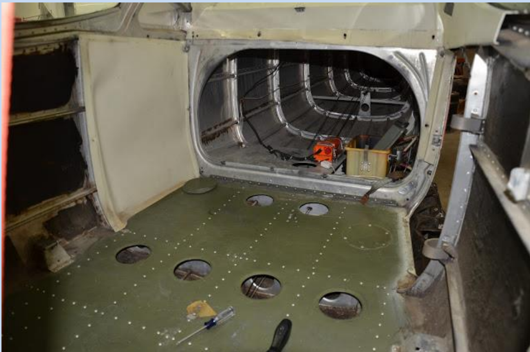
Rear Seats Removed
