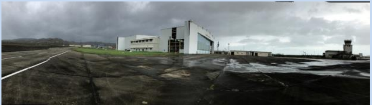
Figure 5 Large hangar building after Maria. Siding is torn off, one of the large rolling doors was blown open, and the aircraft within tossed about. A C172 took flight inside the hangar and was on top of some other airplanes.
